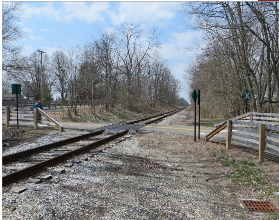
A trail/track crossing on the Camp Chase Trail in Ohio. The trail bends in order to cross the tracks at 90°. (Photo courtesy of the Rails-to-Trails Conservancy)
