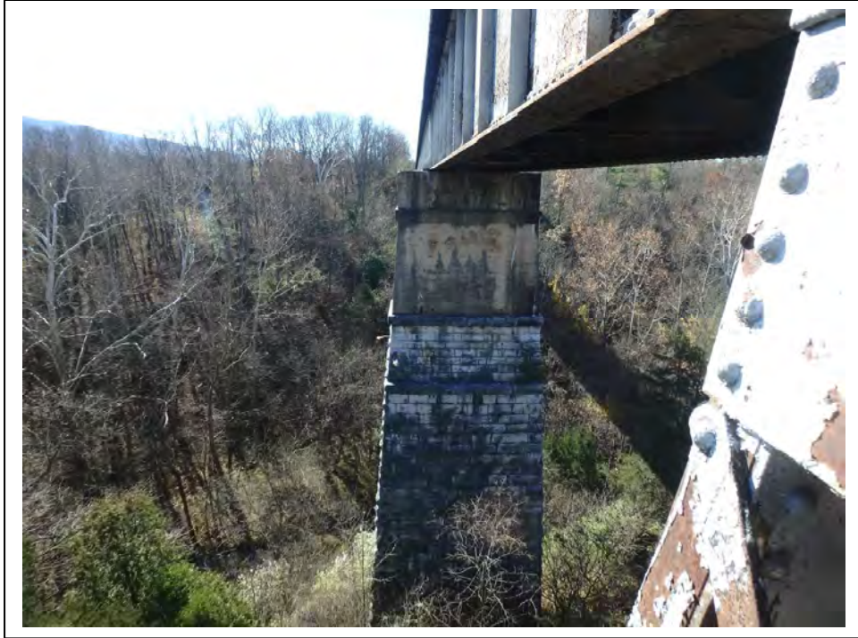
Photo 23: Asset 7643 Pier 7 East Face
