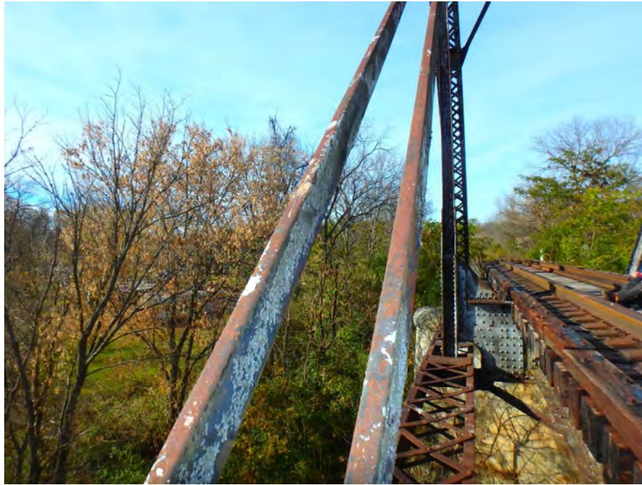
Photo 05: Asset 5104 Span 2/4 Eye-bar Diagonals
