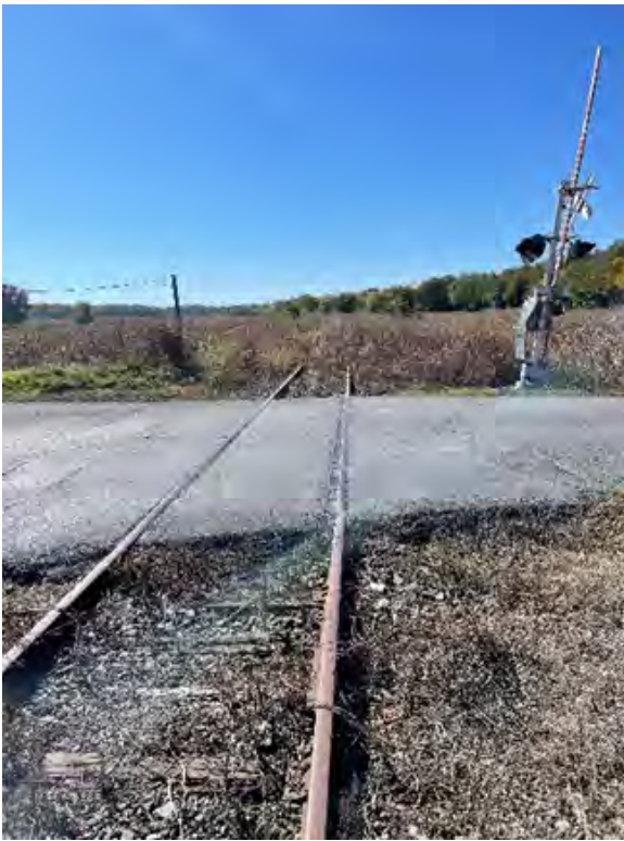
Figure 3 - Evergreen Valley Road Crossing
