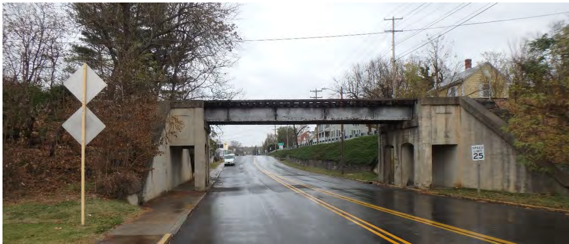
Figure 5. Asset 6141 Overall View
