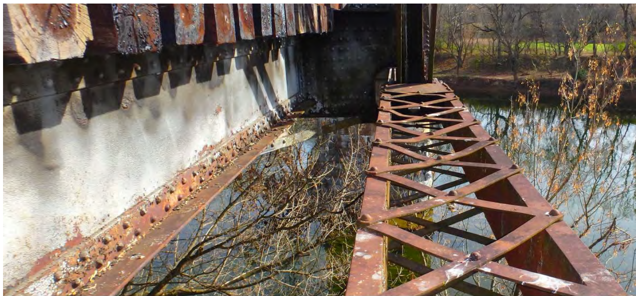
Stringer bolt spacing: 3" Gage, 2.5" Pitch
