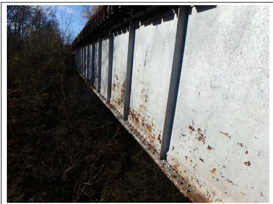
Photo 18: Asset 7643 Span 11 South Face
