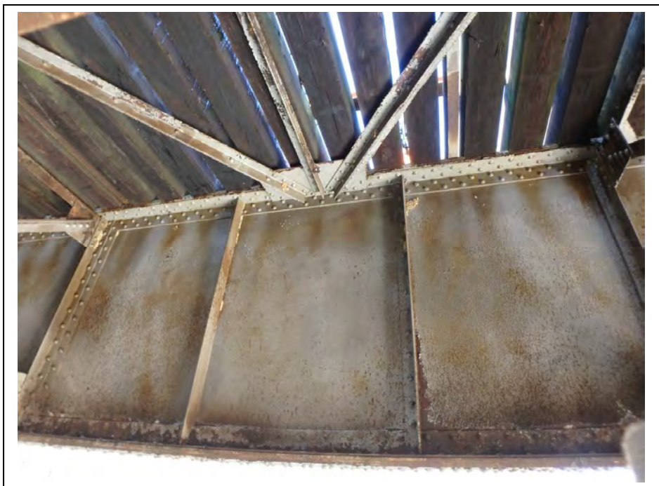
Photo 19: Asset 7643 Span 10 Upper Laterals and Inside Face
