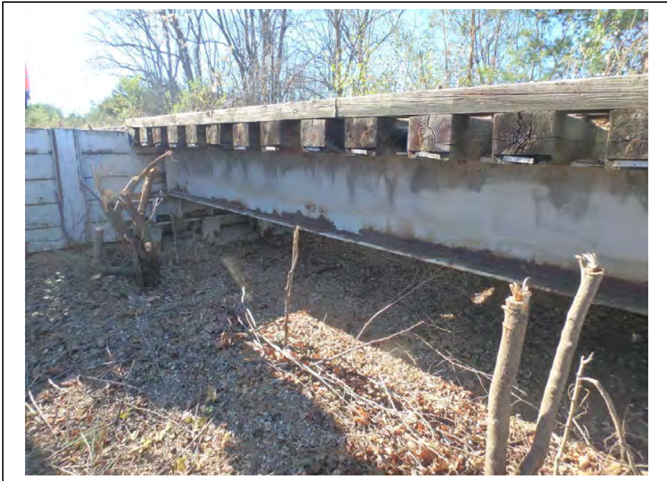
Photo 22: Asset 7643 Jump Span West End
