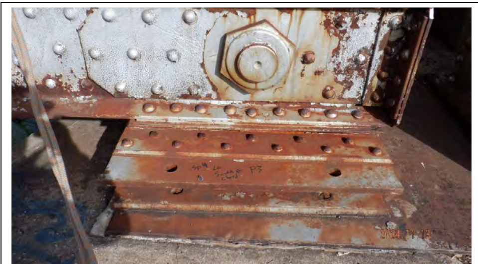
Photo 10: Asset 5104 Span 4 Bearing
