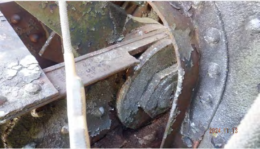
NORTH LOWER CHORD EYEBAR SECTION LOSS (1/4" UP TO 2"?)
