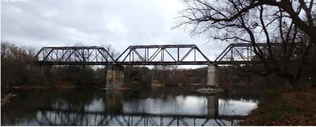
Figure 3. Asset 5104 Overall View
