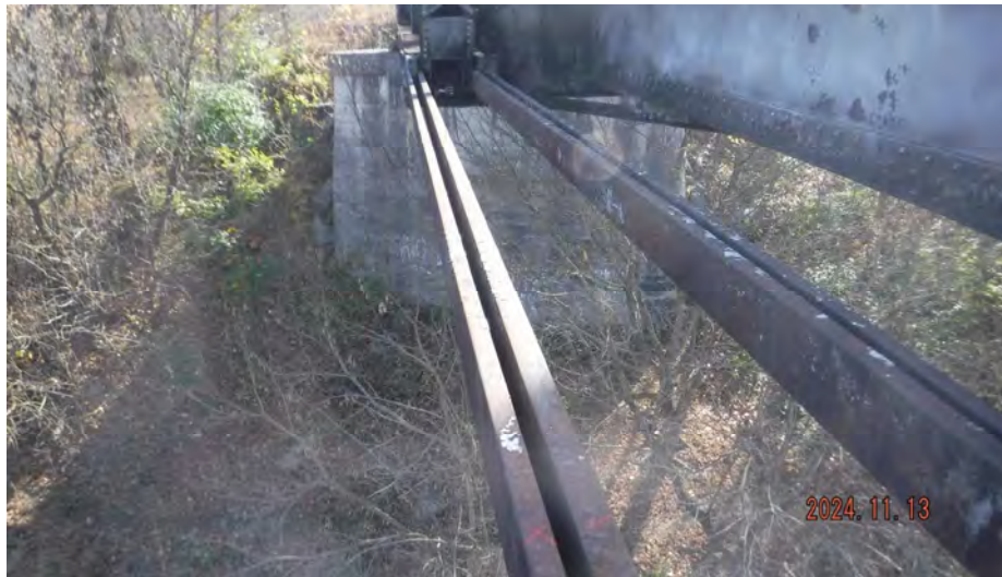
Photo 06: Asset 5104 Span 2/4 Eye-bar Bottom Chord
