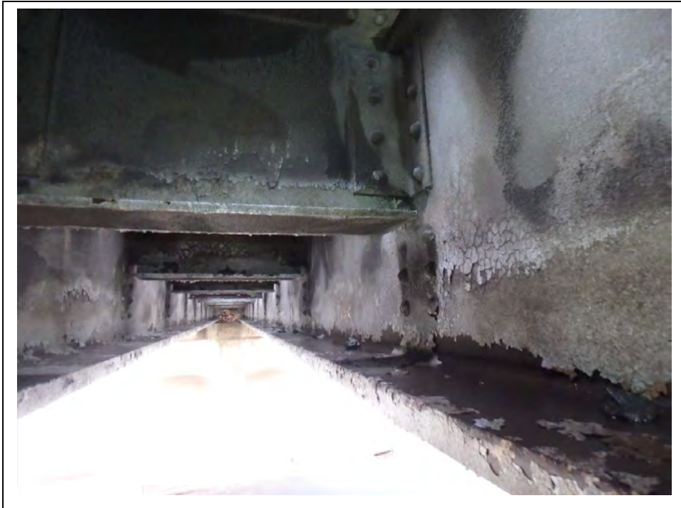
Photo 17: Asset 6141 Diaphragm Connection
