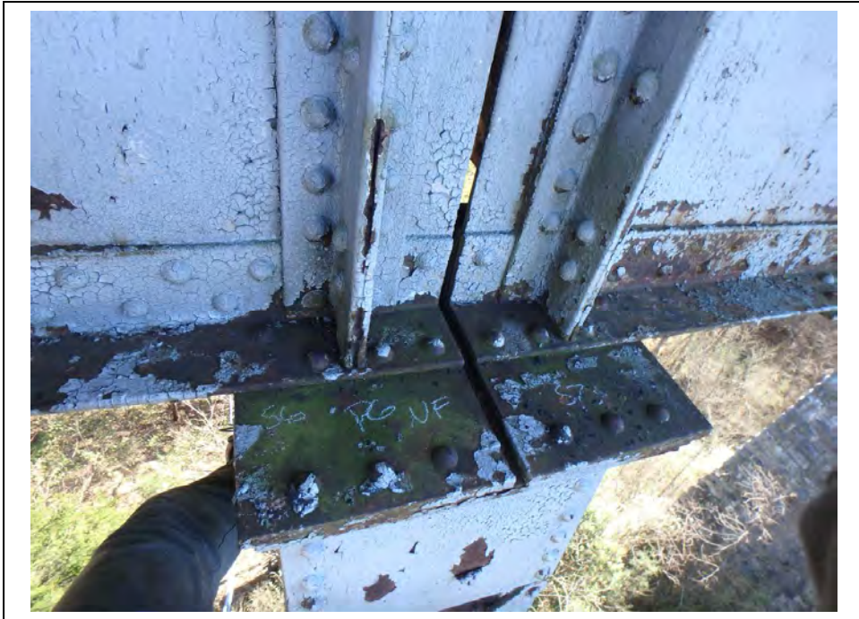
Photo 21: Pier 6 North Face
