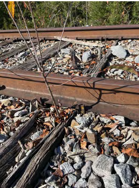
Figure 4 -Defective Crosstie
