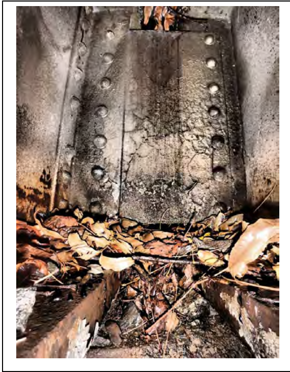
Photo 15: Asset 6141 Diaphragm Connection at Interior Beams
