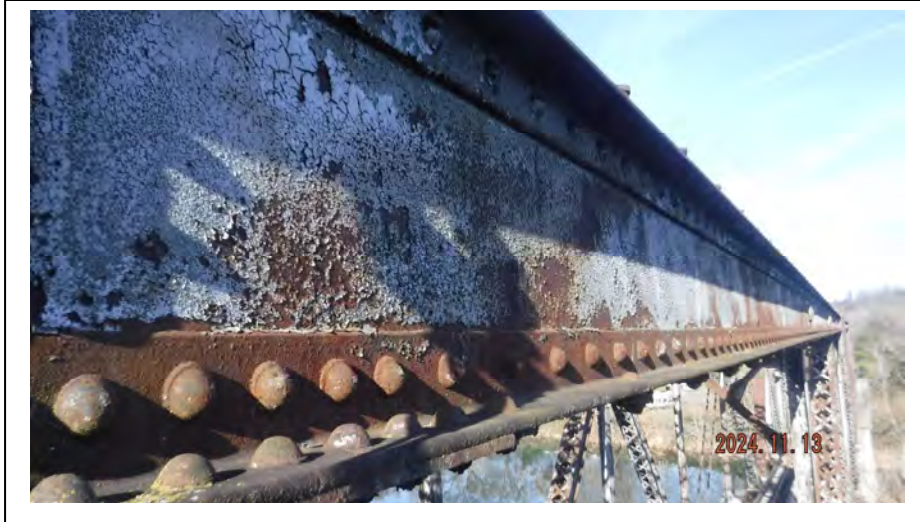
Photo 07: Asset 5104 Span 2/4 Upper Chord
