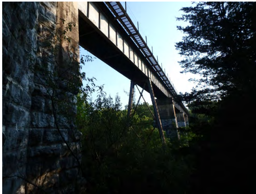
Figure 7. Asset 7643 Overall View
