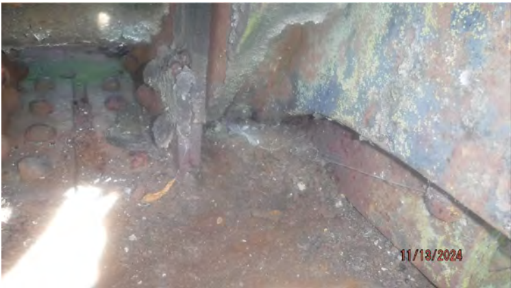
NORTH LOWER CHORD EYEBAR SECTION LOSS (1/4" UP TO 2"?)
