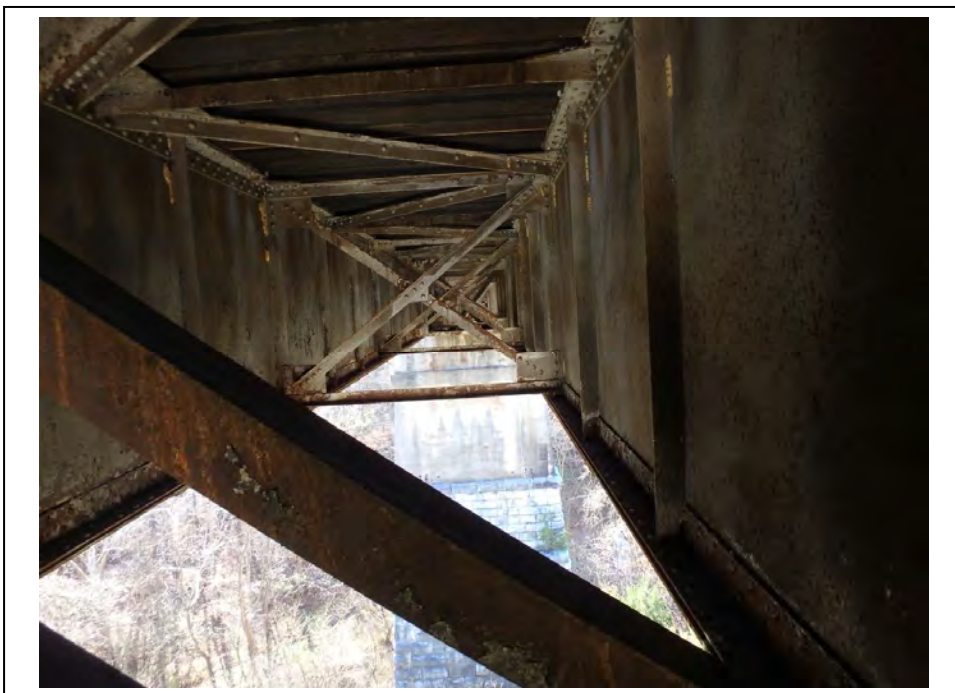
Photo 20: Asset 7643 Span 7 Cross Frames
