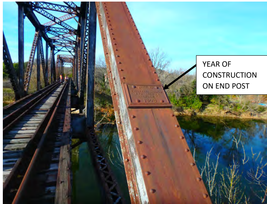
Figure 13. Through Truss Construction Year (Span 3)
