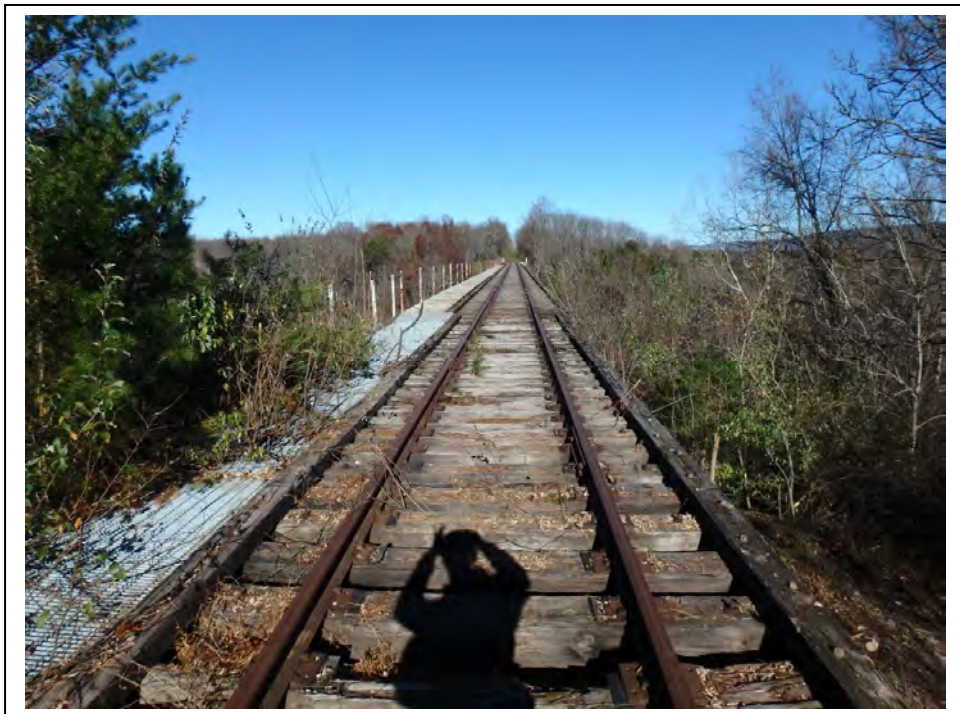
Photo 24: Asset 7643 Track Level
