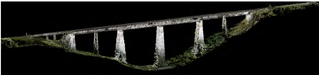
Figure 20. Asset 7643 Scan Data Overall View
