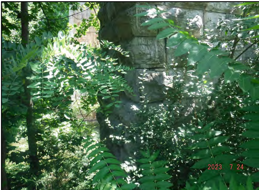
Photo 4: Typical Stone Masonry Portion of Pier
