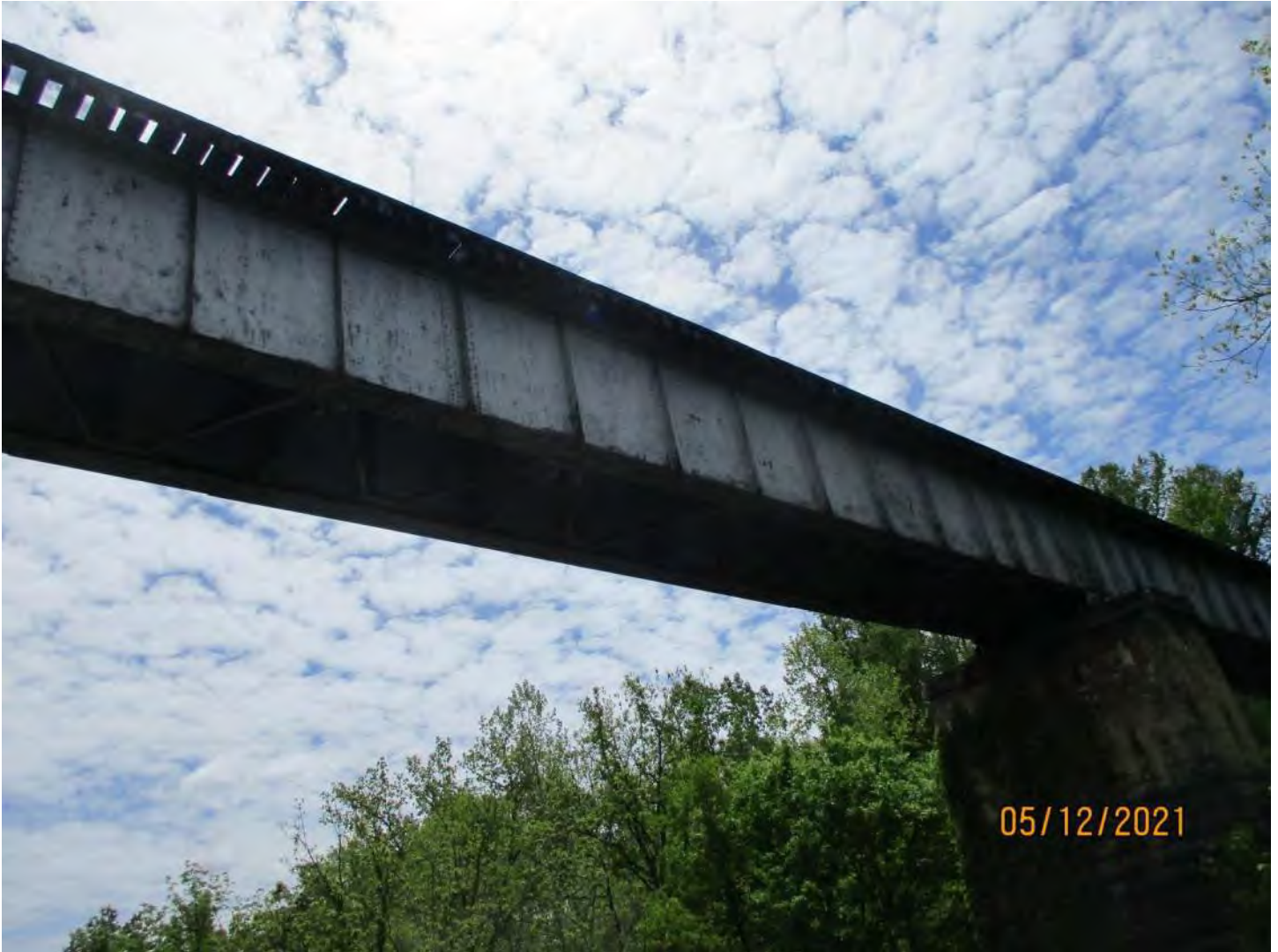
Asset 8627 over North Fork Shenandoah River and Bryce Blvd N 38° 44' 37.22", W 78° 38' 45.09" Three Span Steel Girder Bridge, 425'-0"
