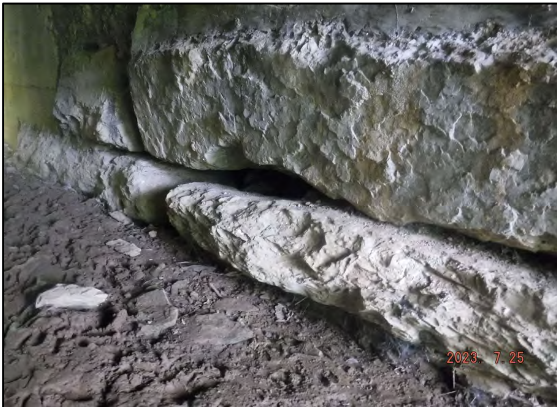
Photo 6: Typical Stone Masonry Abutment Open Joints
