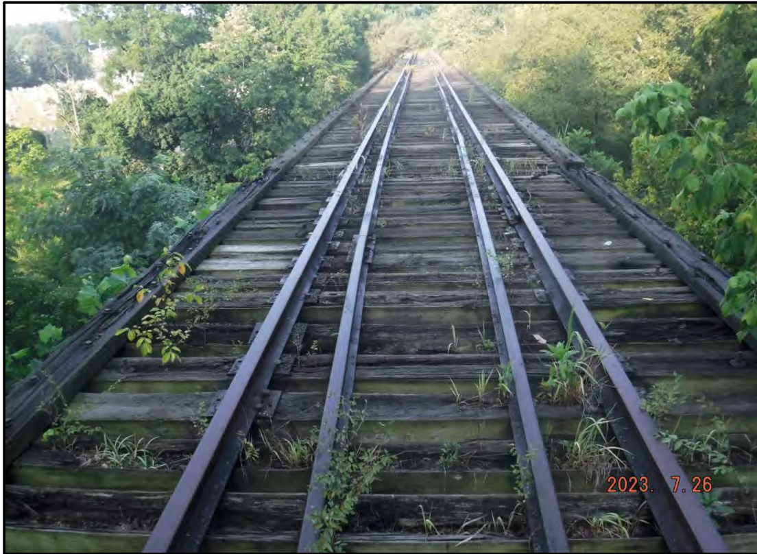
Photo 1: General Condition of Timber Tie Deck
