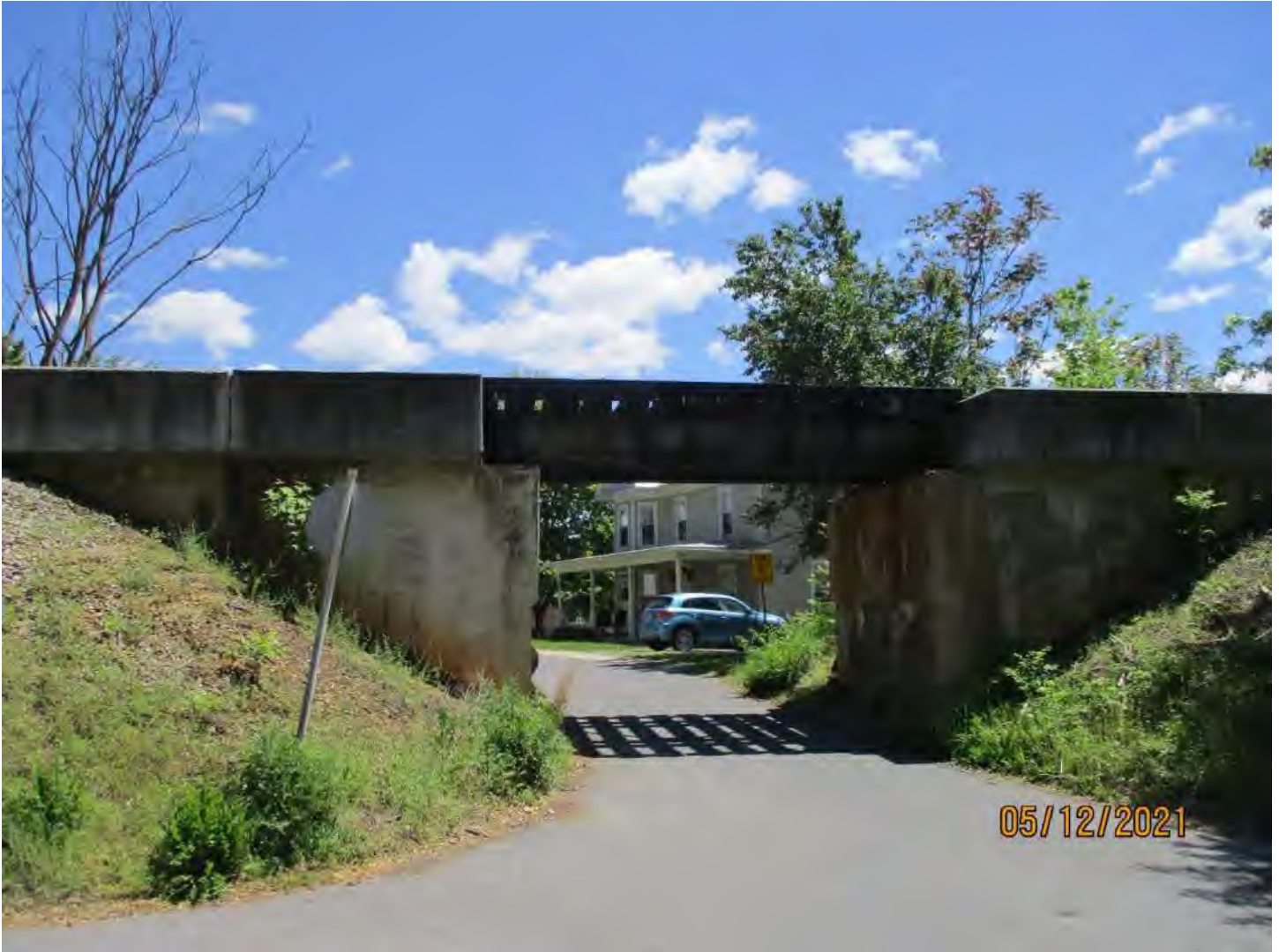
Asset 8620 over Bank Street N 38° 44' 40.55", W 78° 38' 42.92" Single Span Steel Double Girder Unit Bridge, 20'-10"
