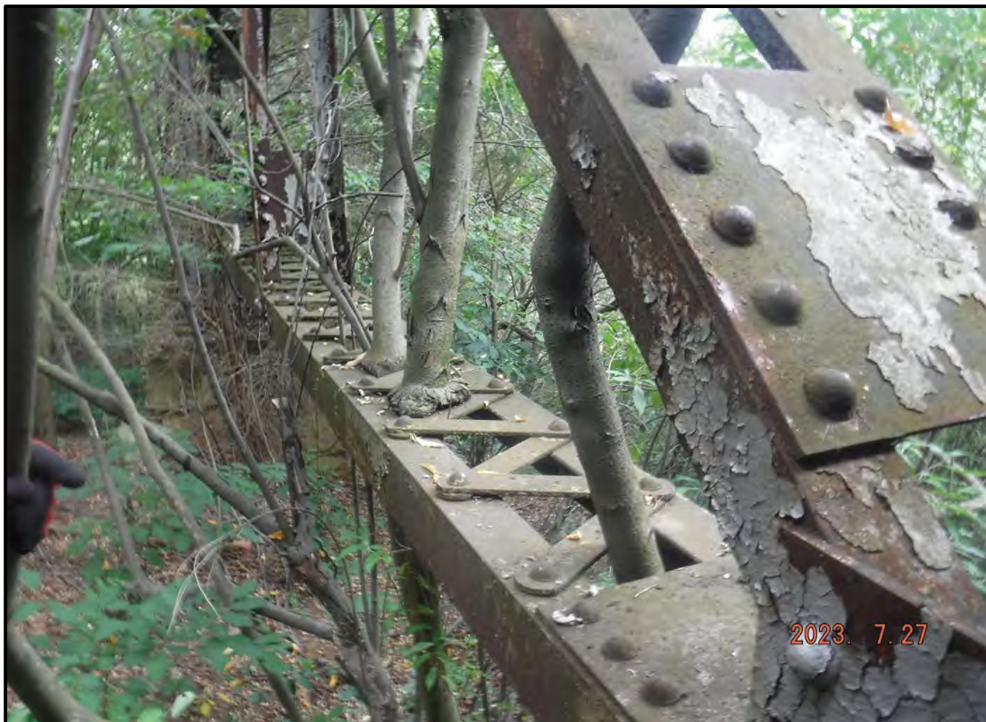
Photo 6: Typical Vegetation in Steel Bent Bracing
