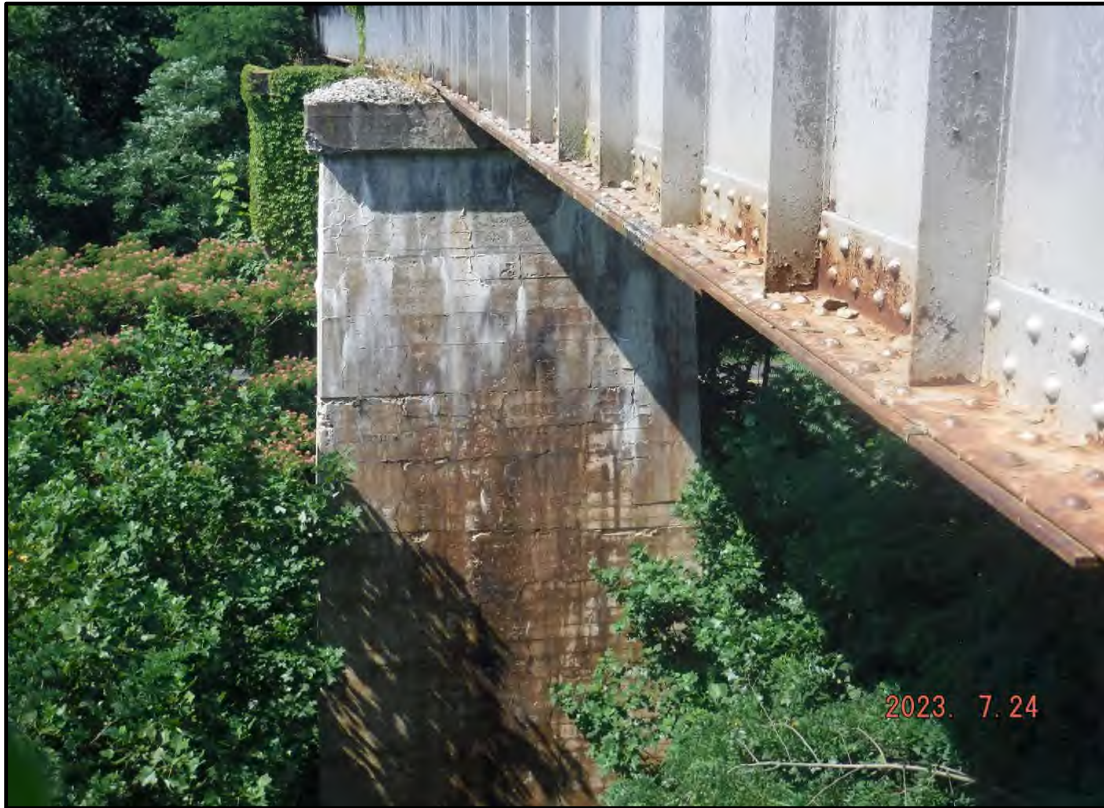
Photo 3: Typical Reinforced Concrete Portion of Pier
