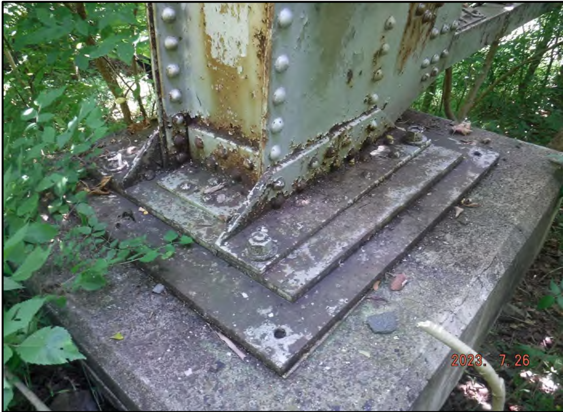
Photo 5: Typical Steel Bent Tower Bearing and Pedestal
