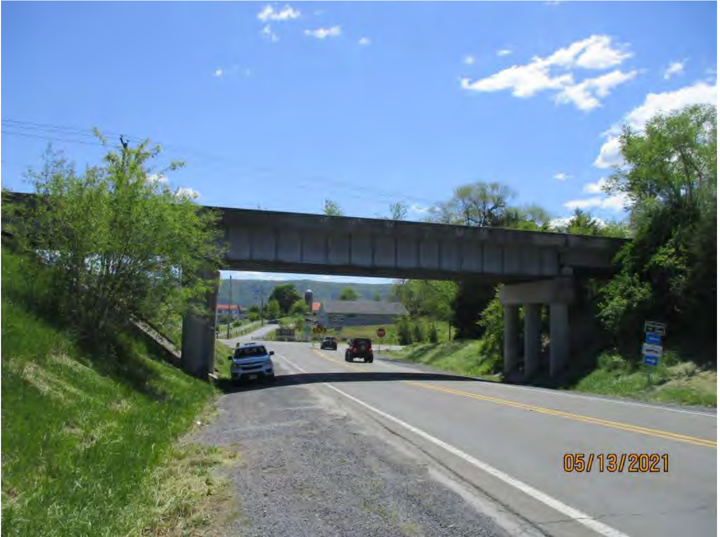
Asset 6669 over Rte 651 Mt Olive Rd N 38° 57' 17.50", W 78° 25' 43.73" Three Span Steel Girder Bridge, 127'-0"
