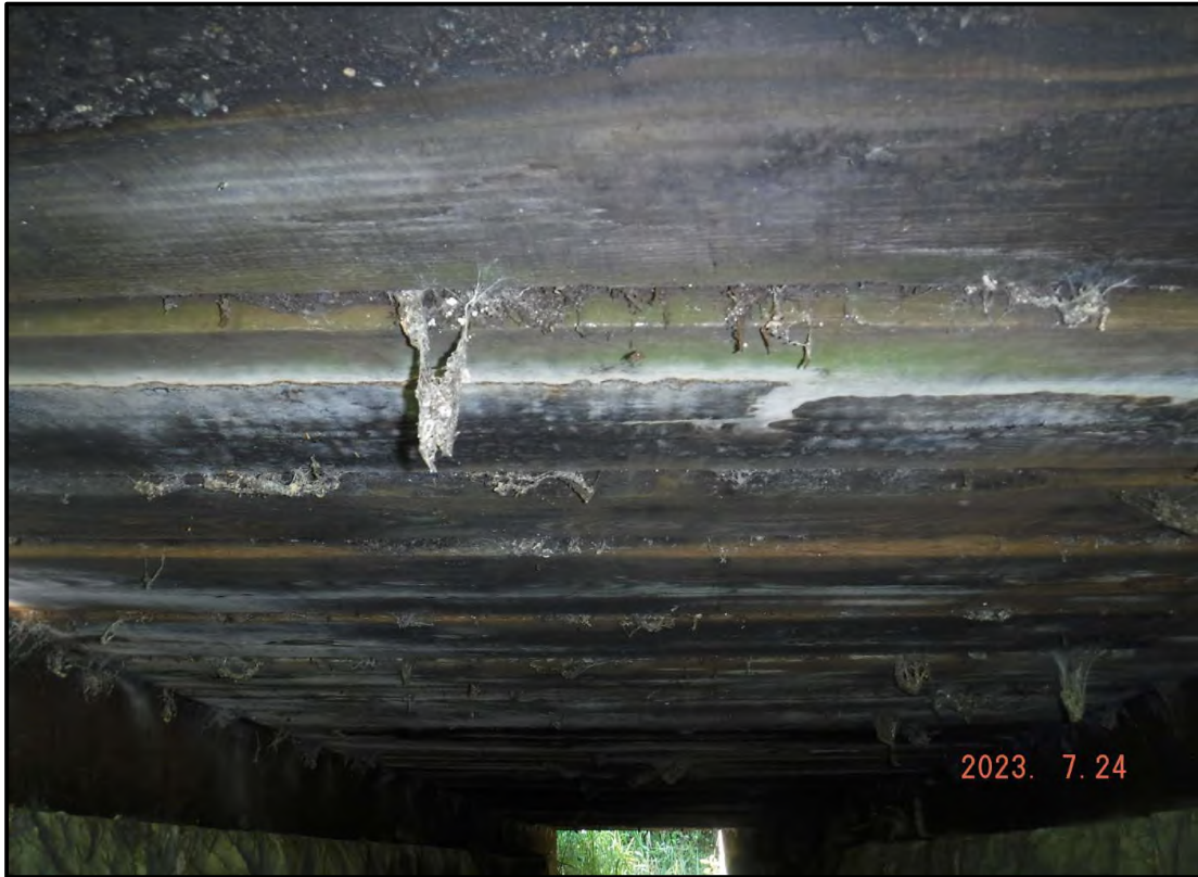
Photo 3: Typical Condition of Timber Slab
