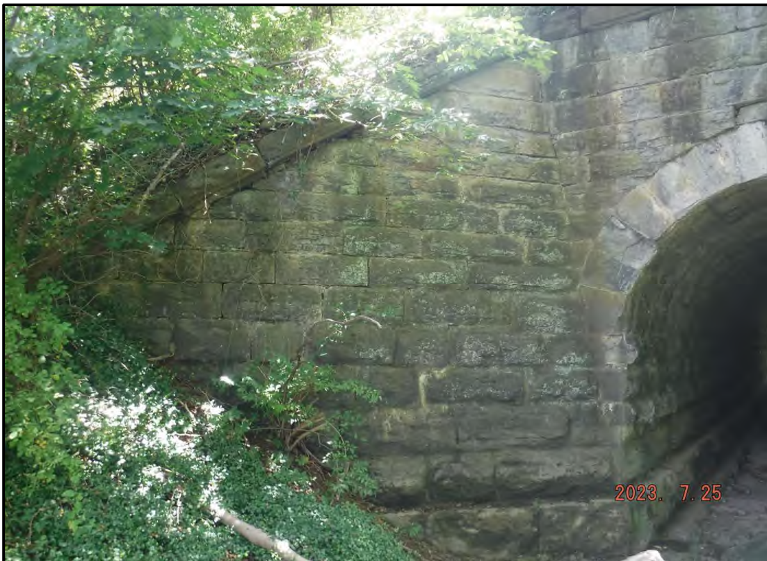
Photo 6: Typical Wingwall (NE Wing Shown)
