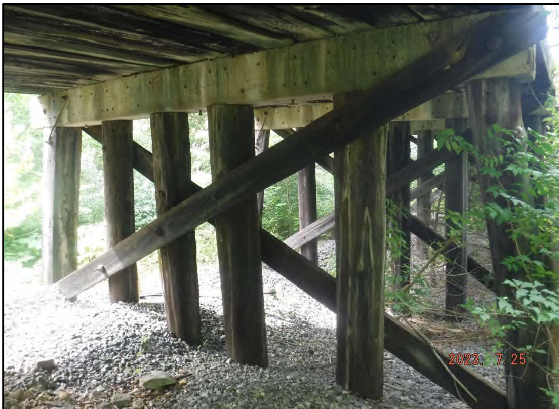
Photo 4: Typical Timber Pile Bent
