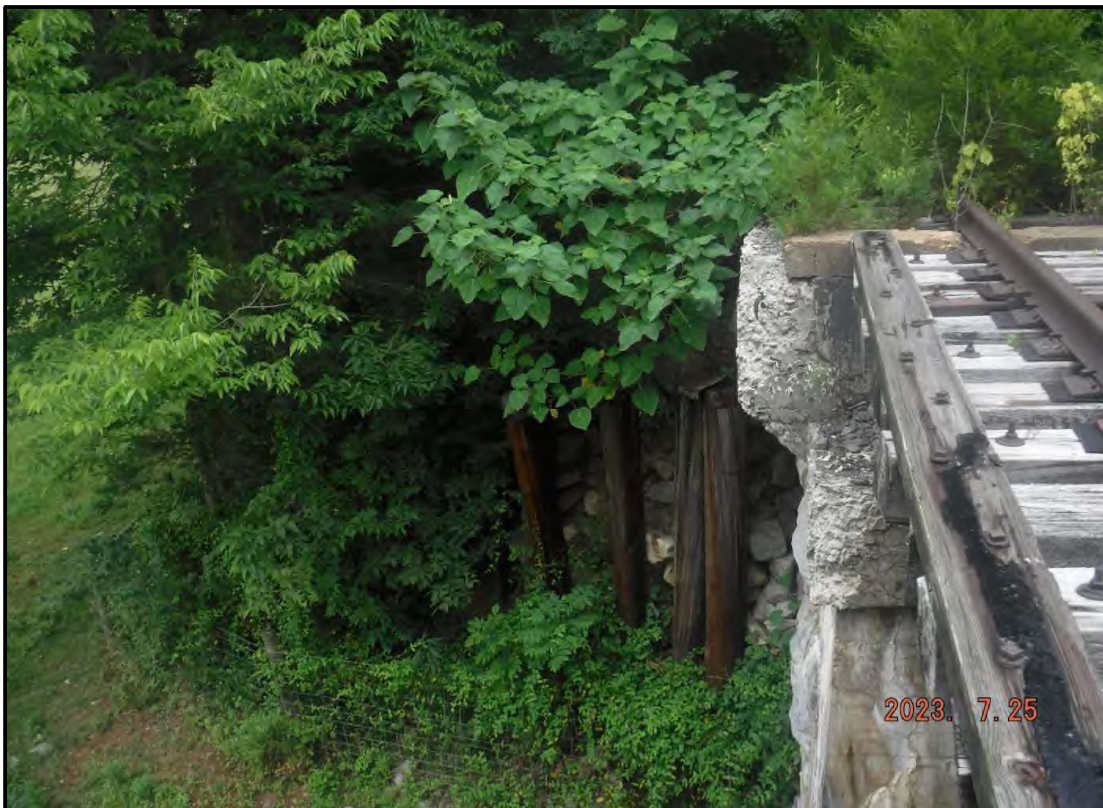
Photo 4: Typical Wingwall (NE Wing Shown)
