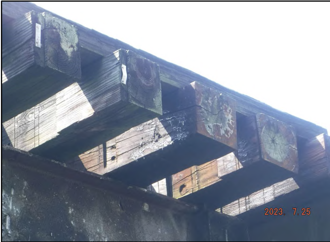
Photo 3: General Condition of Timber Tie Deck
