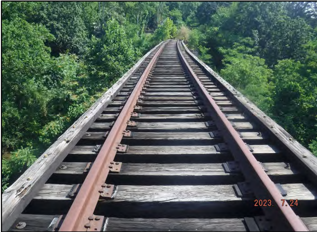
Photo 1: General Condition of Timber Tie Deck
