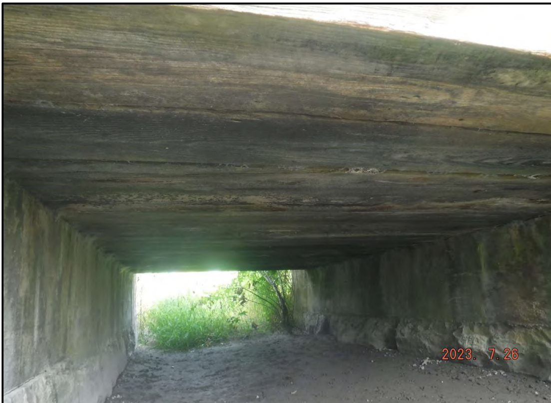
Photo 4: Underside of Timber Slab
