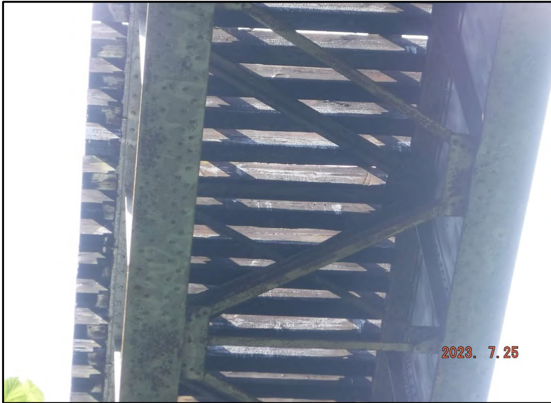
Photo 1: General Condition of Timber Tie Deck
