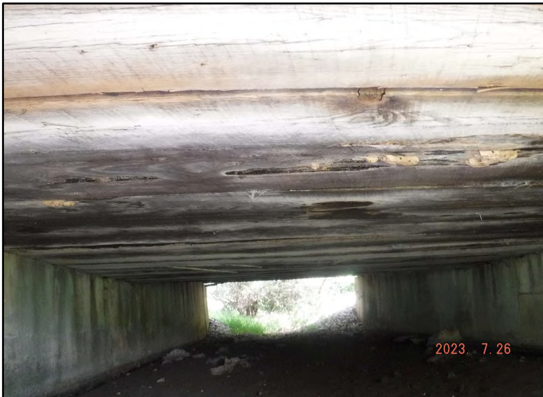
Photo 4: Typical Timber Slab (From North)
