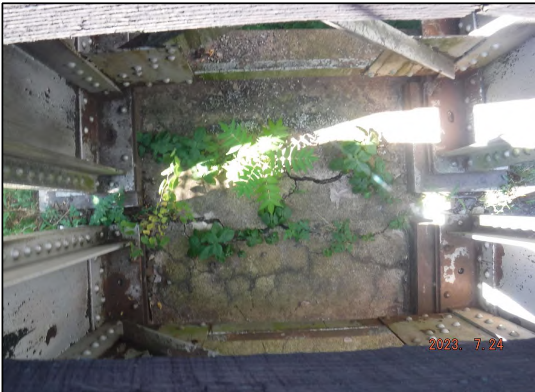
Photo 2: Pier 3 Bridge Seat With Wide Cracks
