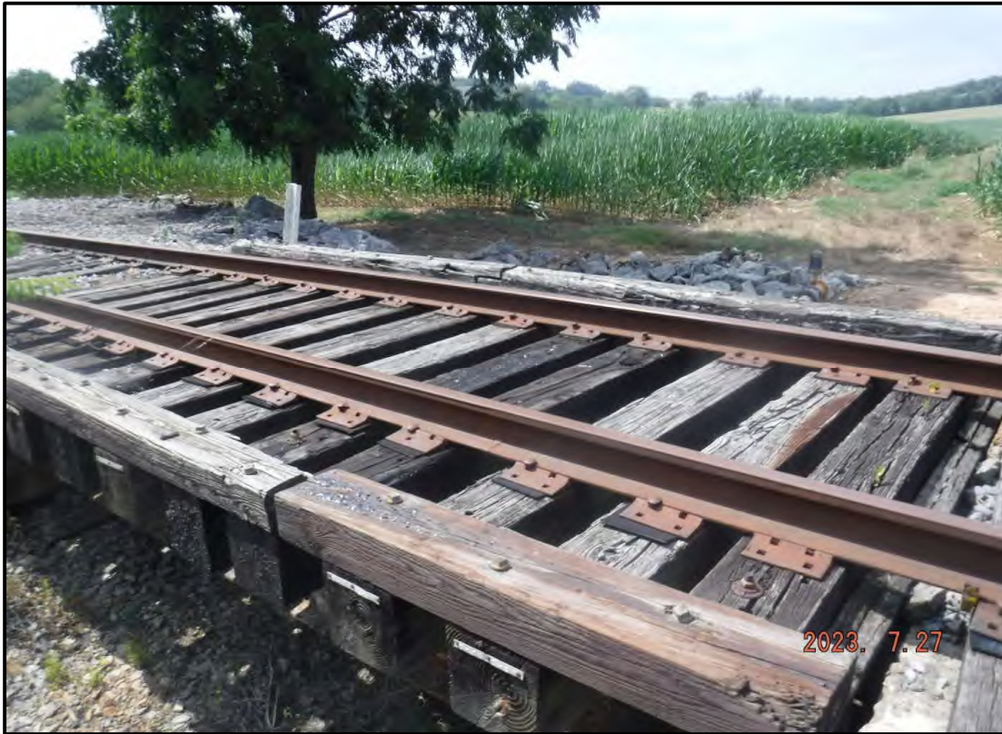
Photo 1: General Condition of Timber Tie Deck
