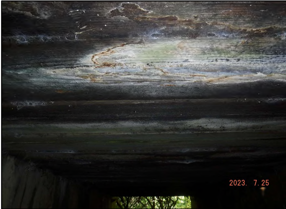
Photo 5: Typical Underside of Timber Slab
