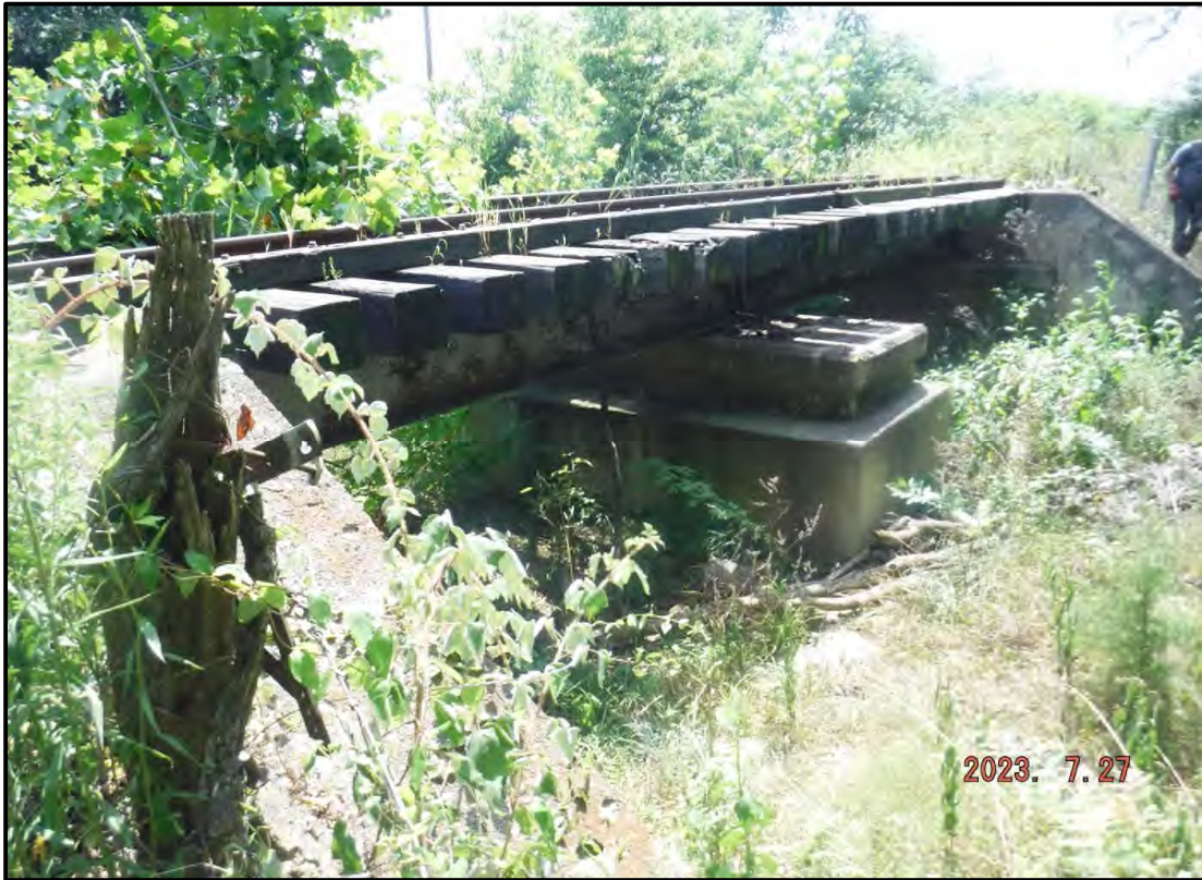
Photo 1: General Condition of Timber Tie Deck
