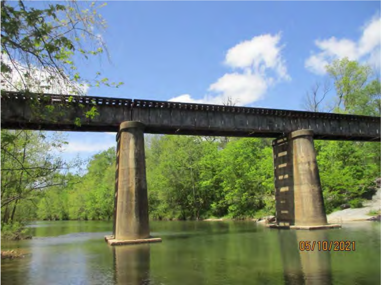
Asset 9970 over North Fork Shenandoah River N 38° 38' 11.38", W 78° 46' 51.59" Four Span Steel Girder Bridge, 184'-0"
