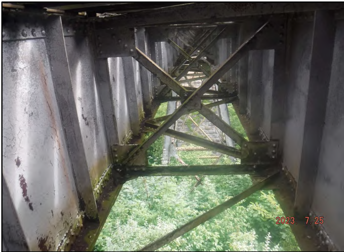
Photo 3: Through Girders (From West Abutment)
