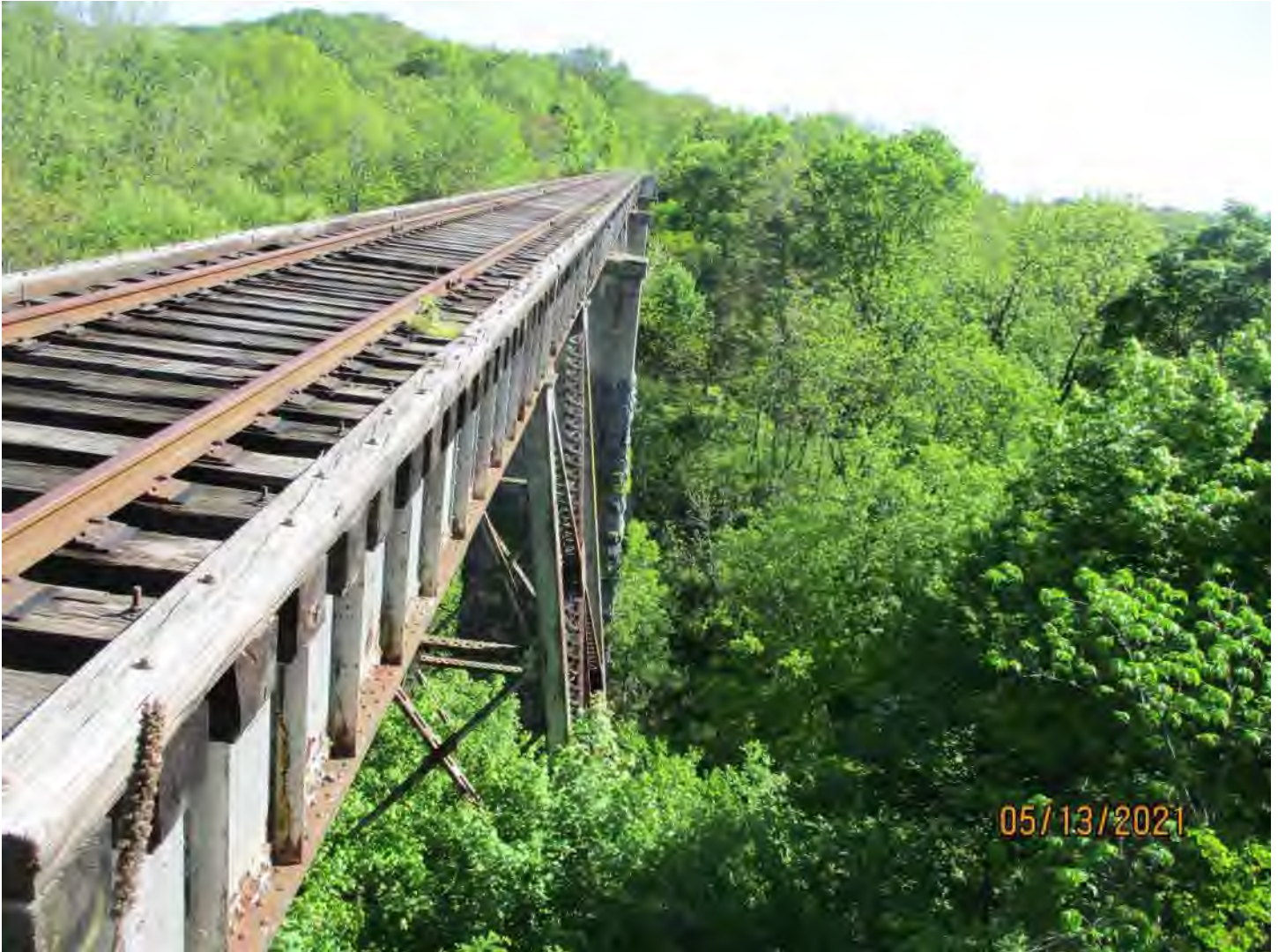
Asset 7164 over Pughs Run N 38° 54' 12.88", W 78° 29' 24.81" Nine Span Steel Two Girder Bridge, 380'-0"
