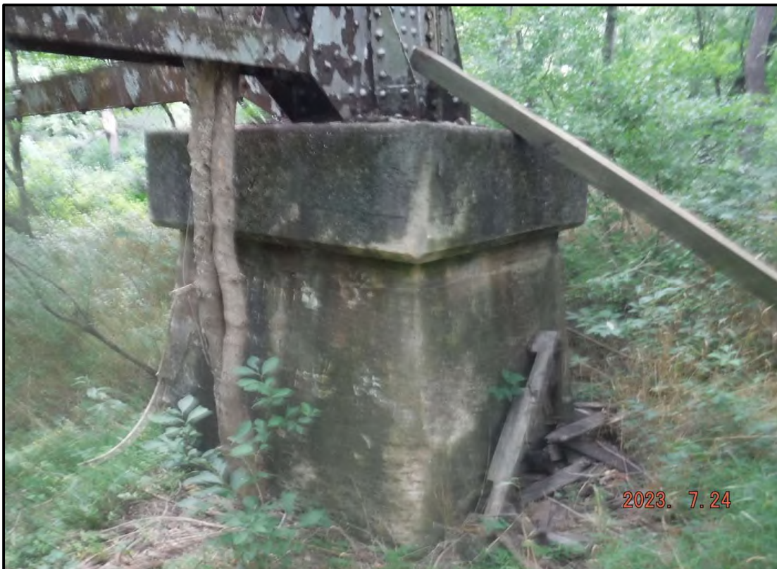
Photo 4: Typical Steel Bent Tower Pedestal
