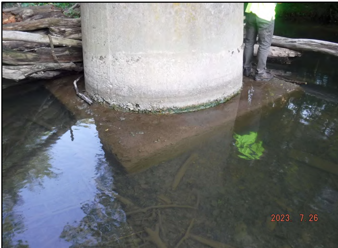
Photo 6: Typical Exposed Footing (Steel Bent Tower)
