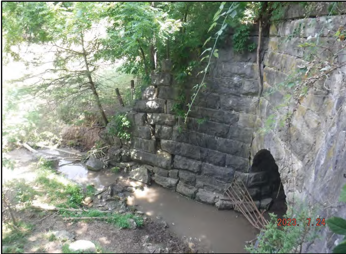
Photo 5: NE Wing with Free End Separation
