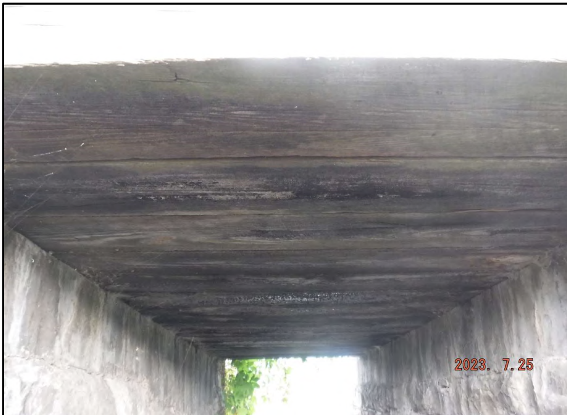
Photo 4: Underside of Timber Slab
