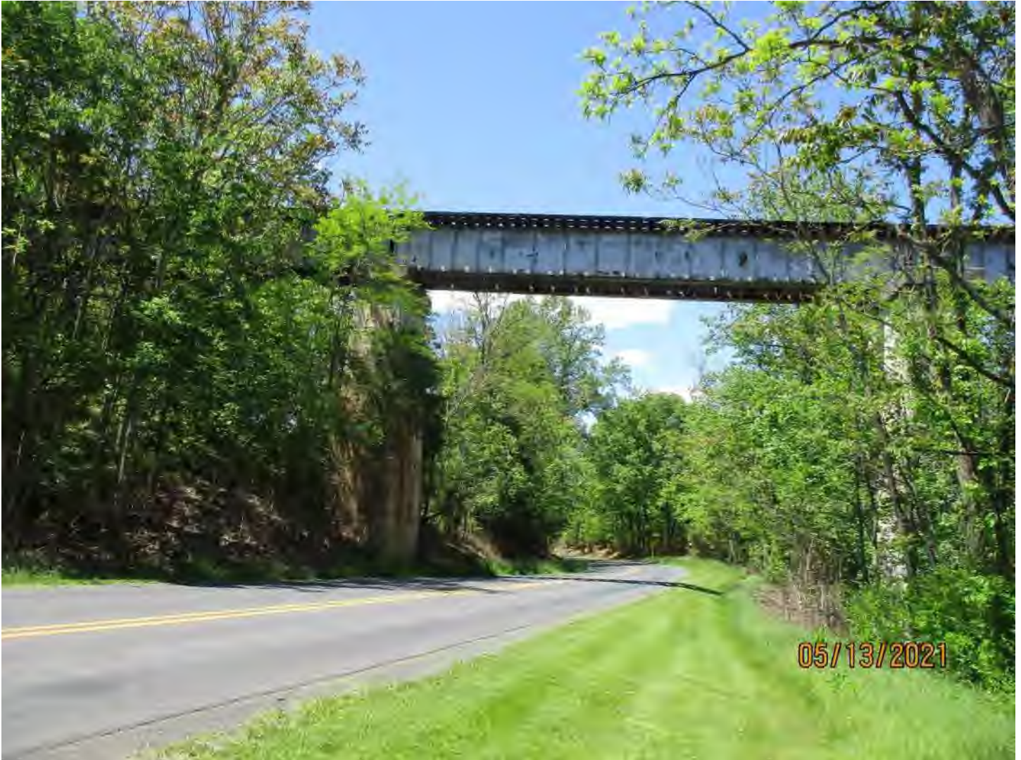
Asset 6391 over Battlefield Rd and Tumbling Run N 38° 59' 3.73", W 78° 23' 50.09" Four Span Steel Two Girder Bridge, 262'-0"
