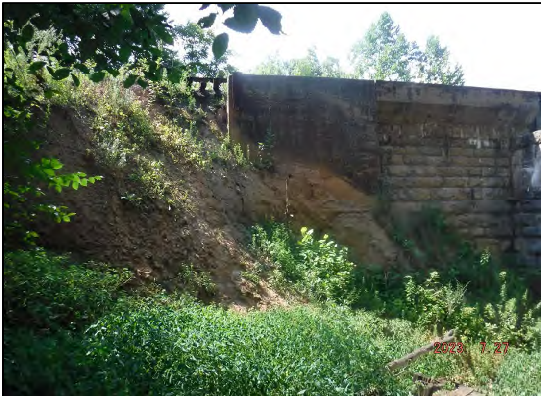
Photo 2: Erosion/Washout at SW Corner of Structure
