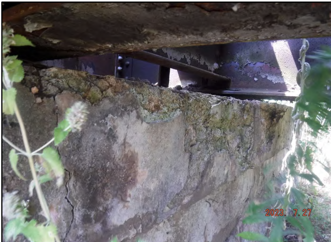
Photo 6: Typical Spalled Bridge Seat (Outside of Bearings)
