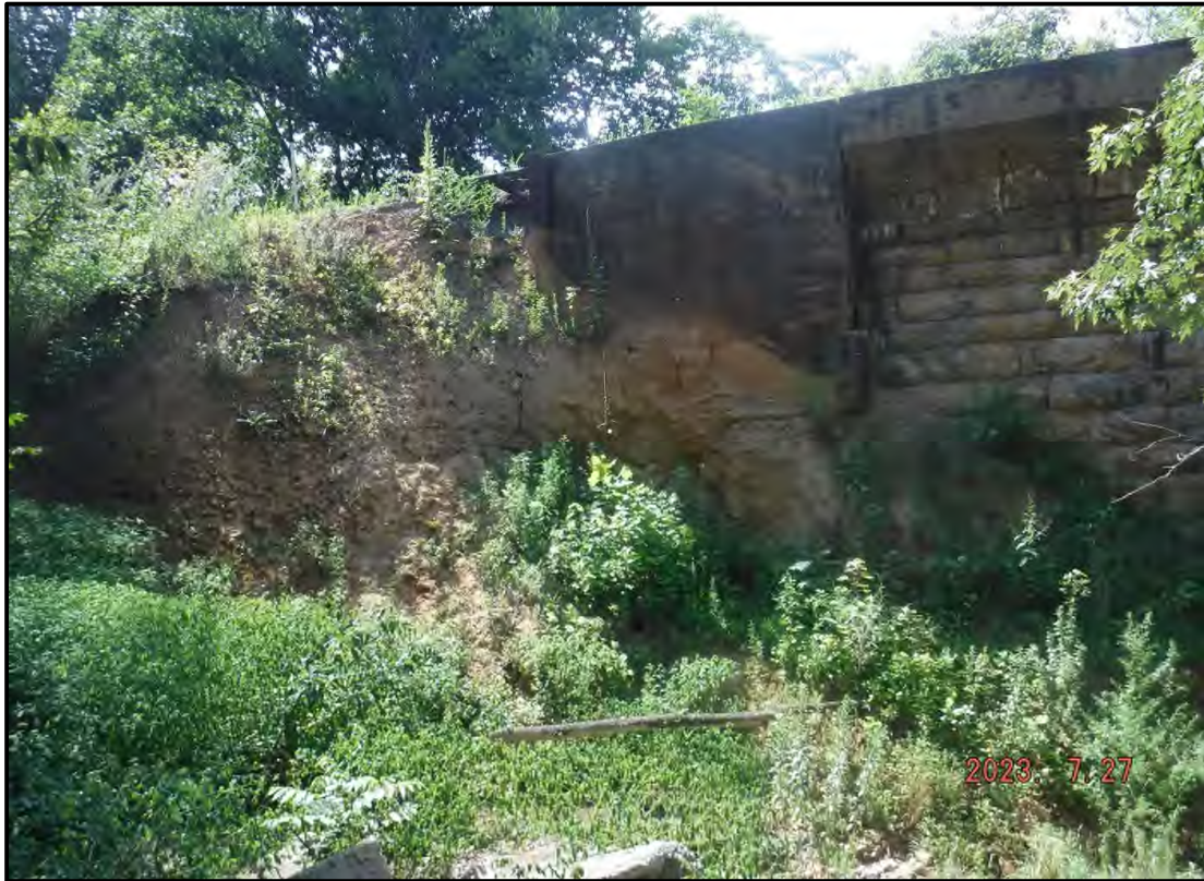
Photo 1: Erosion/Washout at SW Corner of Structure
