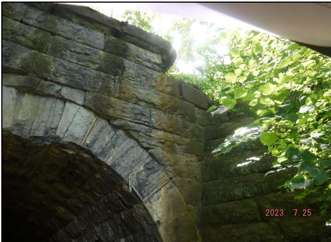
Photo 2: Missing Stones West End of North Headwall
