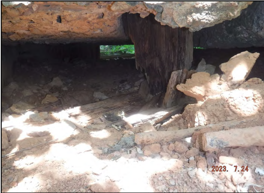
Photo 5: Undermined East Approach Ballast Trough
