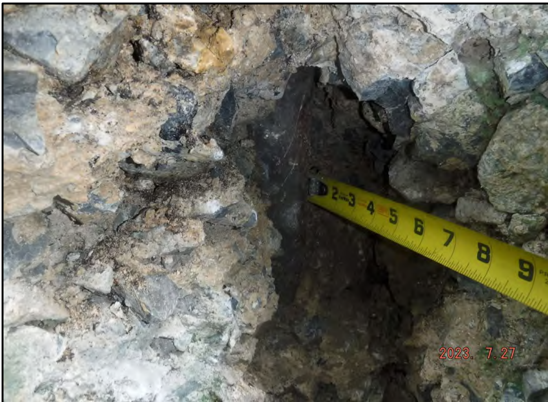
Photo 8: Spalled Concrete on Main Span Bent 2 North Pedestal
