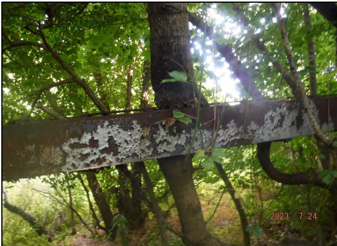
Photo 2: Vegetation Growth in Steel Bent Tower Bracing
