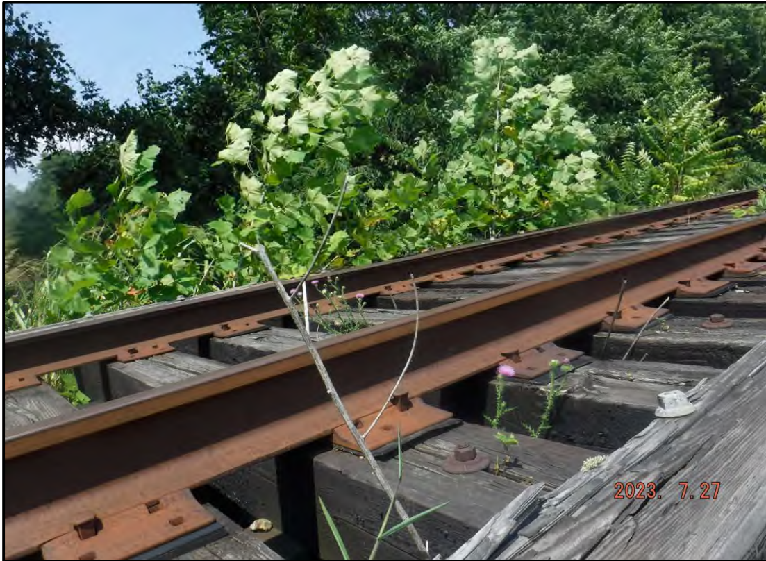
Photo 1: General Condition of Timber Tie Deck
